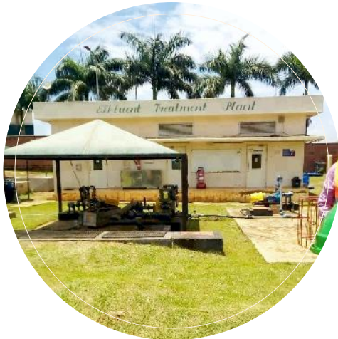
Effluent treatment plant
