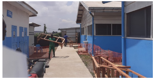
A side view of the Djoungolo CTC during the handover of central logistics cholera kits (cholera beds, IV poles, pools tester, beacons, sprayers, Jerrycans) by WHO: on the left, the health personnel ward and, on the right, the cholera patient hospitalization rooms.
