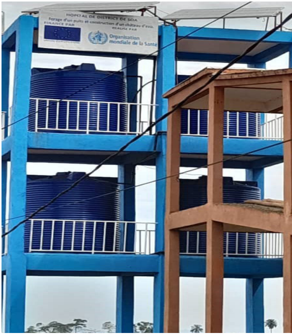
Photo. Borehole/water tower in Soa 90%completion
