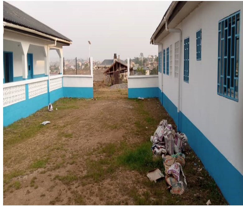
Photo. CMA Olembe rehabiliation at 80%
