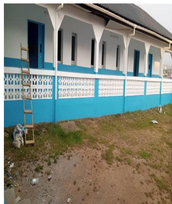
CMA Olembe 100% completed rehabilitated on April, 2023
