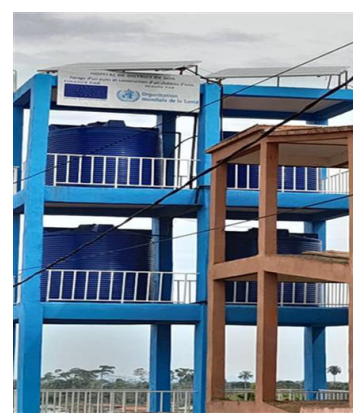
Borehole and watertower in Soa tower 100% completed rehabilitated on April, 2023
