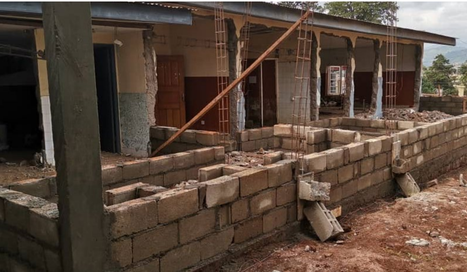
Photo : Bamenda intensive care unit (ICU) during construction
