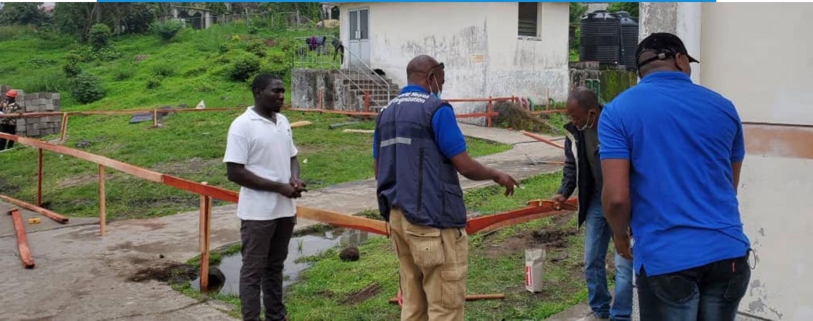
Photo : Buea Intensive care unit (ICU) before construction
