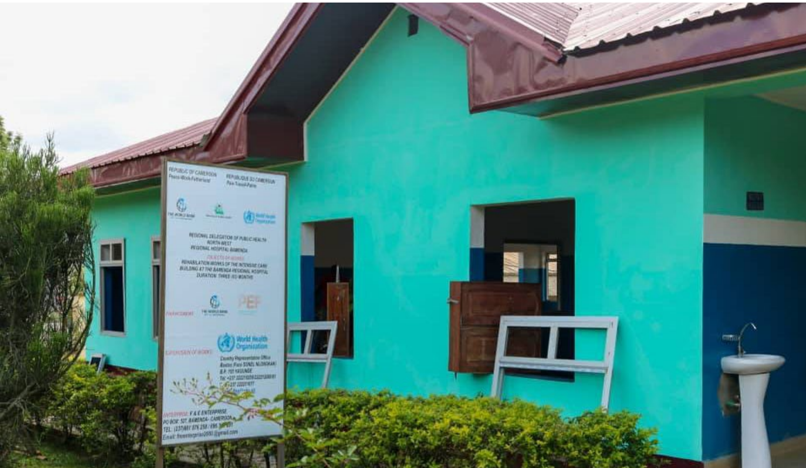
Photo : The rehabilitated intensive care unit (ICU) of Bamenda
