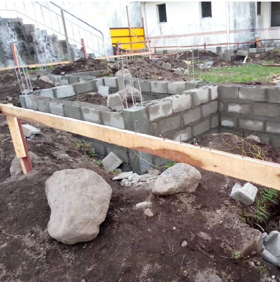
Photo : Buea intensive care unit (ICU) during construction
