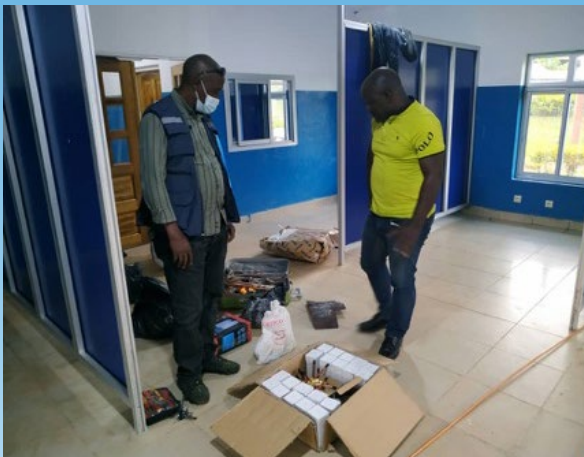
Installation of an oxygen supply system in the intensive care unit (North-West Region)
